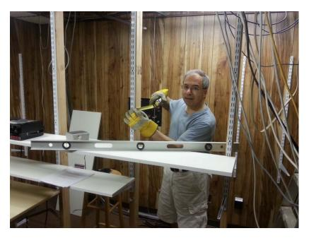
The 2' x 4' frame was constructed such that the spacing between the vertical studs was precisely the spacing I needed to accommodate the radio and the PC monitors I intended to use. Before I began construction, I made several trips to Micro Center, measuring monitor heights, widths, and lengths – finally settling on 21.5" Dell LED monitors and designing the 2' x 4' stud spacing appropriately.
