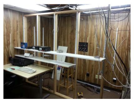
The right-most of the five vertical studs forming the 2' x 4' frame was secured with the plastic-coated deck screws to a floor joist of the room above, through the suspended ceiling, as seen in this photo:
